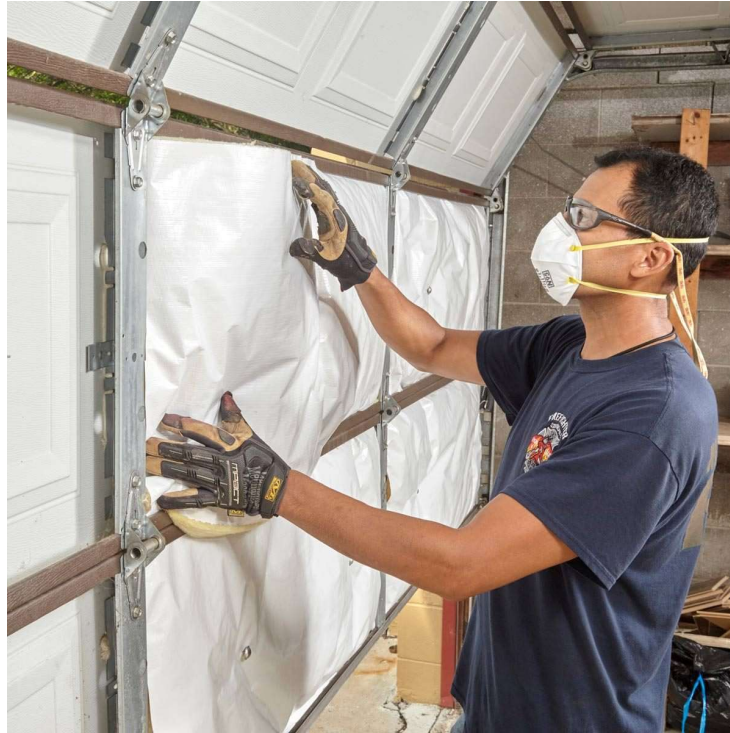
Fig. 11. Home Installation of a Garage Door Insulation Kit, Adapted from [6]
